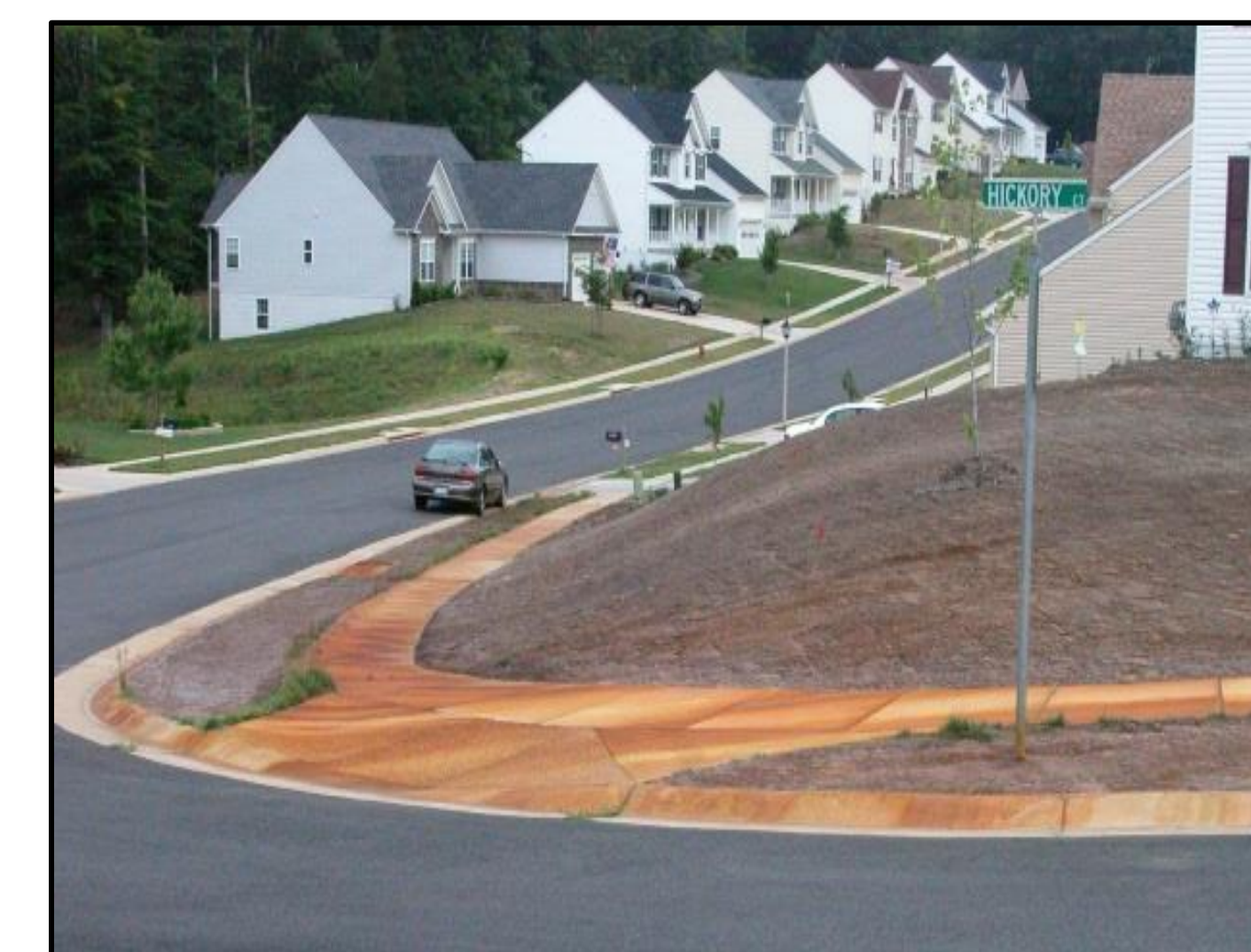
Active acid sulfate soils in Great Oaks development, Fredericksburg, VA. Sidewalks turned red from oxidation and hydrolysis of iron is seepage waters released by oxidation of iron sulfides in soil exposed by excavation.
